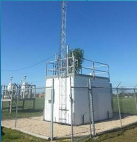
Quapaw's Criteria Pollutant Shelter Site with ammonia monitoring.
